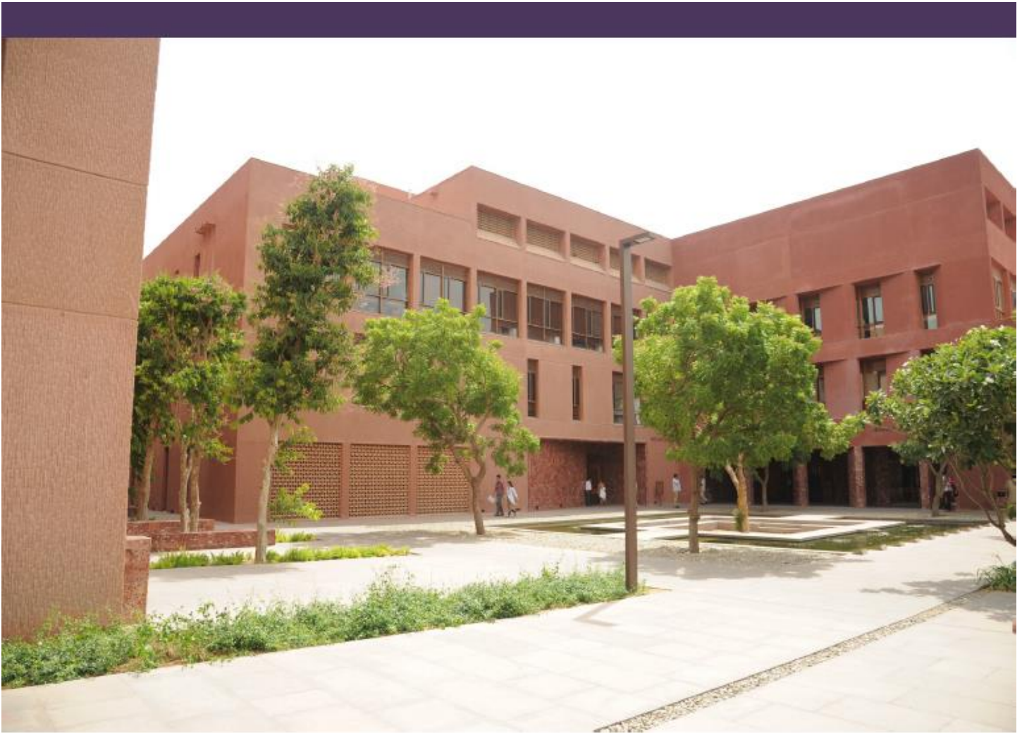
The Ambulatory Care Zone at the Aga Khan University Hospital
